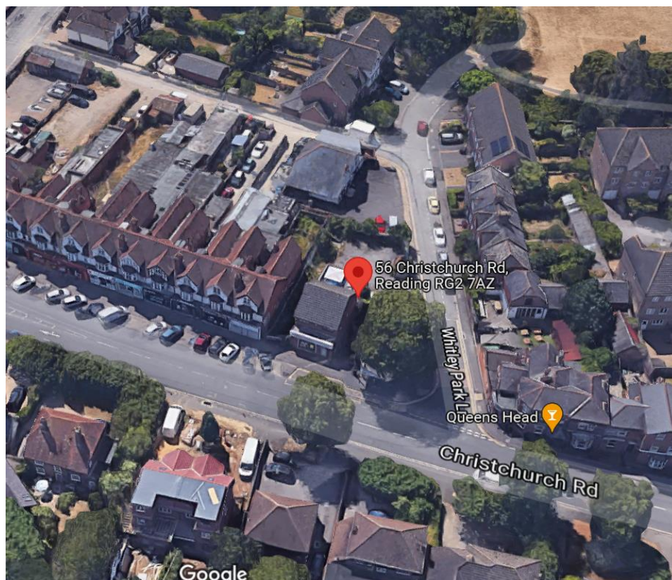
Aerial view of site
